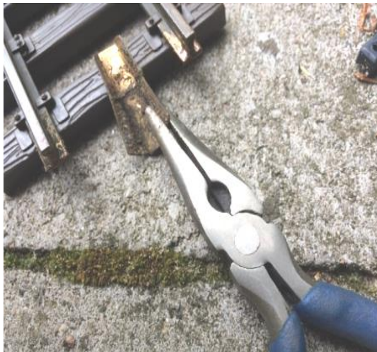
Fig.2.5-15 The contamination accumulated in the rail connector is clearly visible here
